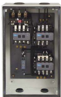
Interior View of MU FASD
