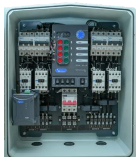
Interior View of xMU-GiA
